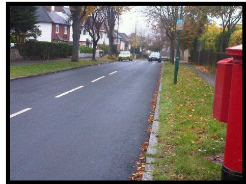
Figure 3.15.3a -This photo depicts a recently resurfaced urban road in good condition
