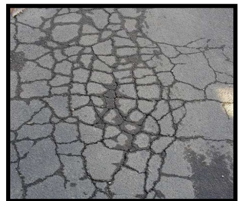
Figure 3.15.3c – Increased cracking
