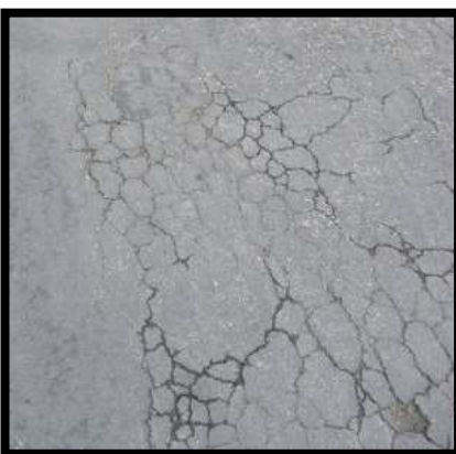
Figure 3.15.3b – Surface cracking
